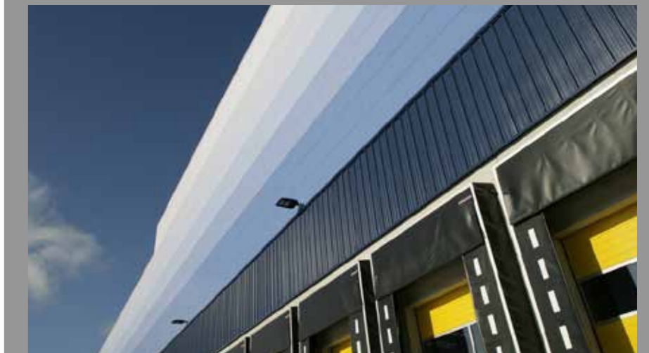
Distribution centre for Waitrose in Milton Keynes using Kingspan products.
