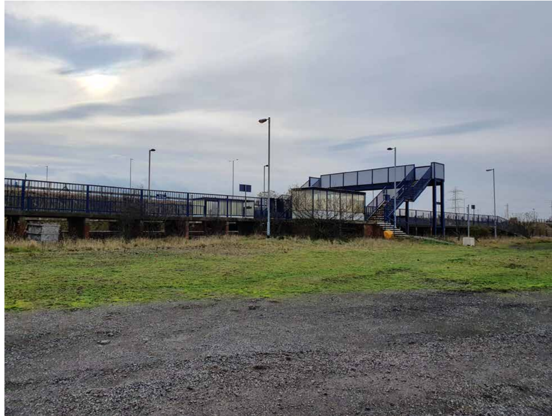
Redcar British Steel Railway Station
